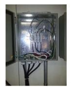
An individual ground wire for each SFTP and CQD shall be run and terminated in the copper ground bus at power junction box at CC Rack location.
