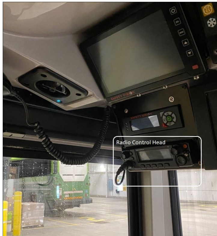
Figure 7: Radio control head location
