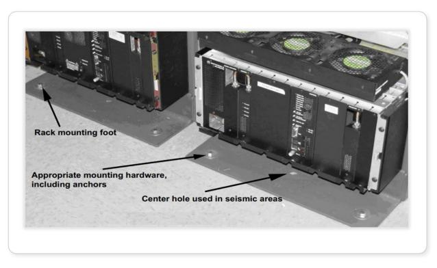
Figure 17: Anchor installation
