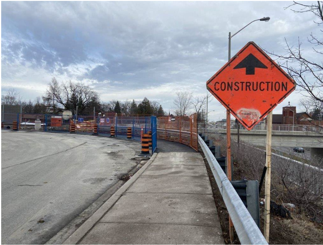
Photo 5: Temporary walkway delineated from roadway with fencing
