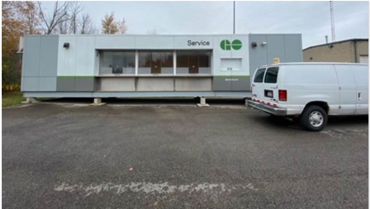
Photo 11: Example of acceptable portable ticket booth - access route to ticket counters not yet installed
