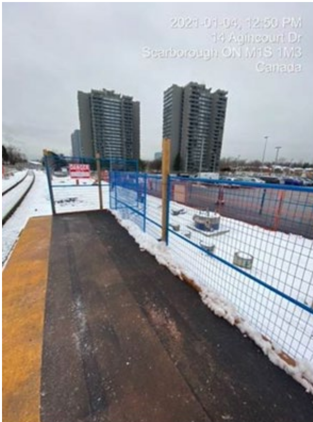
Photo 10: Temporary mini platform with non-slip coating
