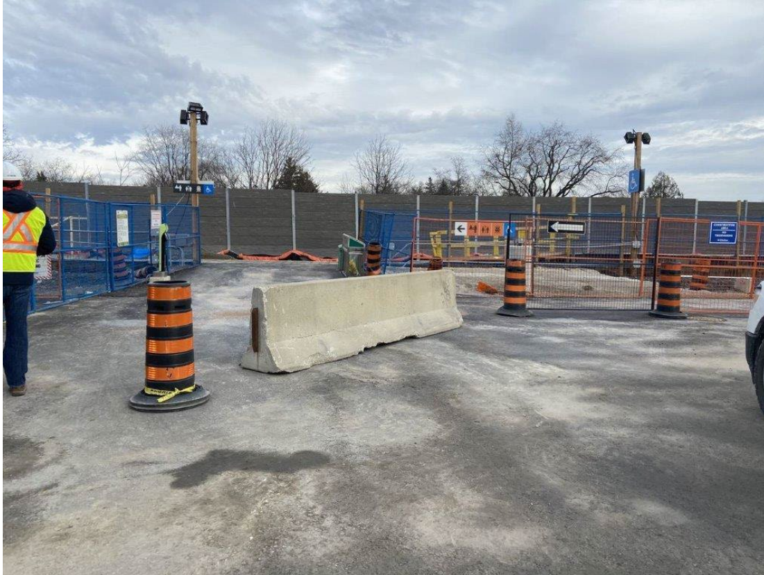
Photo 7: Concrete barrier installed to prevent vehicles entering the temporary walkway
