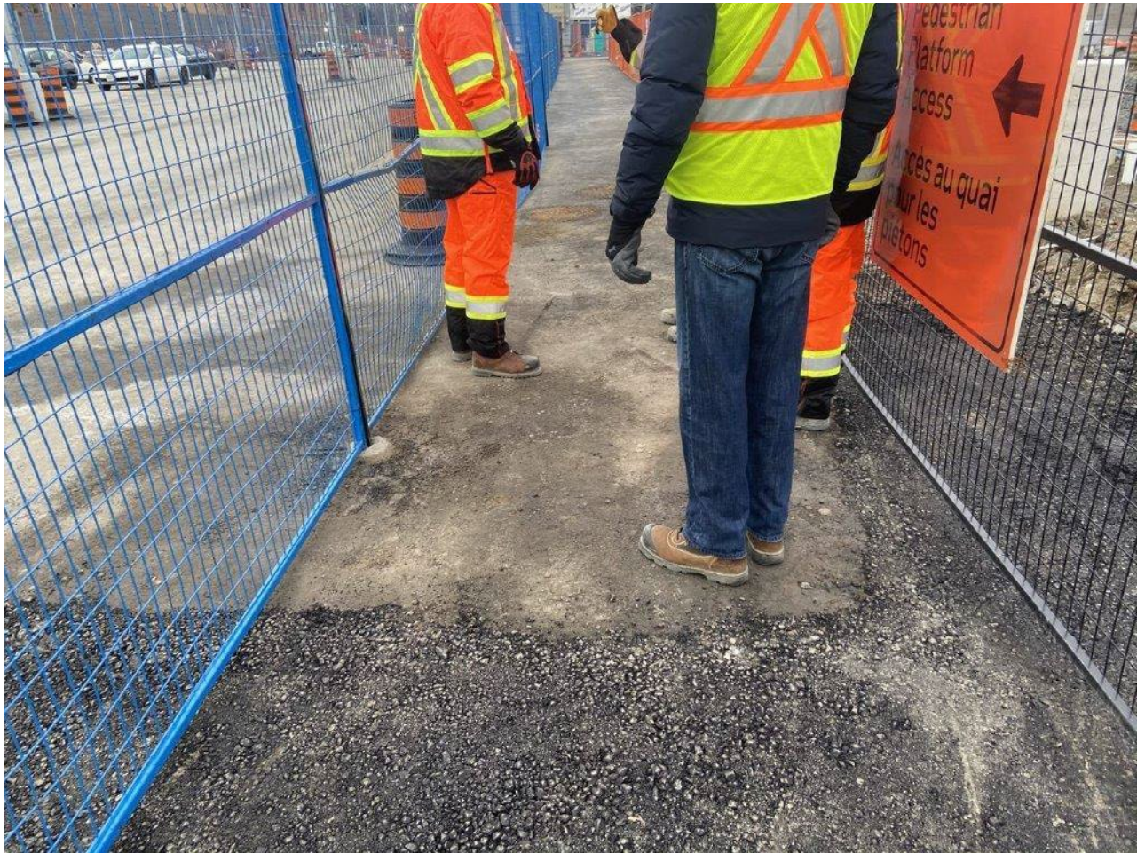
Photo 1: 1800mm clear walkway, fence anchoring prevents tripping hazards
