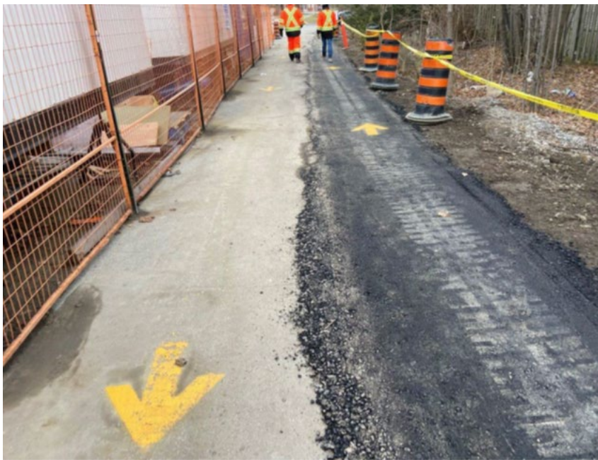
Photo 6: Temporary walkway widened to 1800mm
